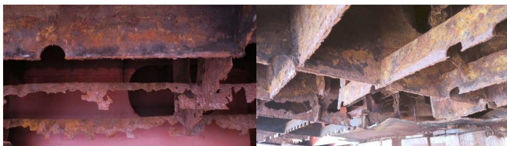
Figure 3.18 Ship in advance stage of corrosion, the resistance structure being severely affected
