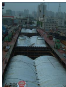
Fig.2-6 Tanc de marfă independent tip C (Lovstad, 2008 17 )
