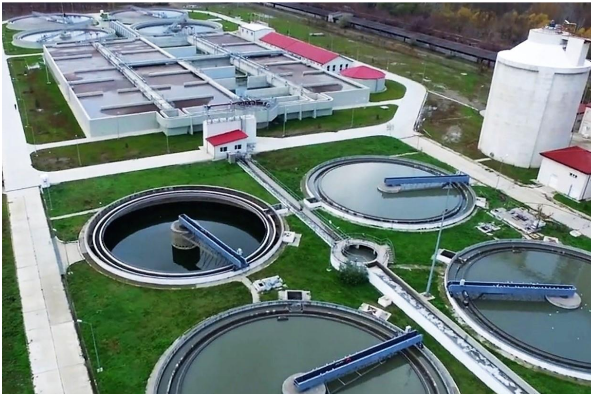
Fig. 2.1 – Overview of the Galati Wastewater Treatment Plant [75]
