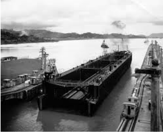
Figure. 1.6. The floating dock ARD-1 constructive version from 1934 [21]
