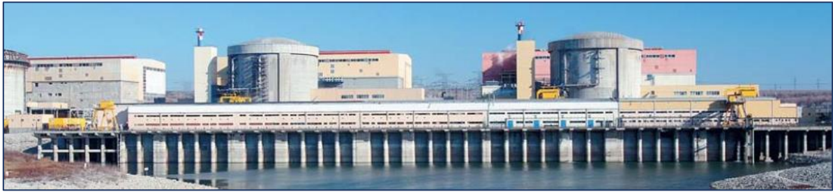
Figure 33 Cernavodă Nuclearoelectric Power Plant (Nuclearelectrica, 2014)
