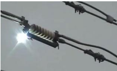
Fig.5.11. The frame selected at the time of stopping of video transmission
